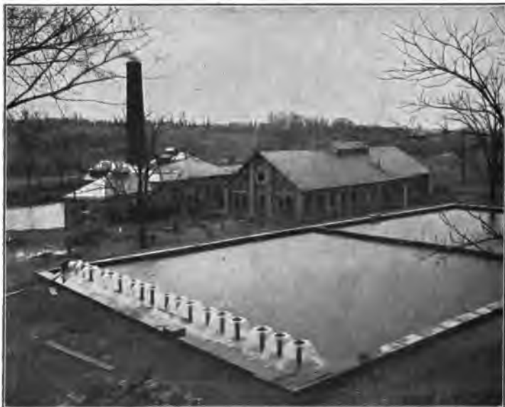
FIG. 46.—Purification of water by aëration.
